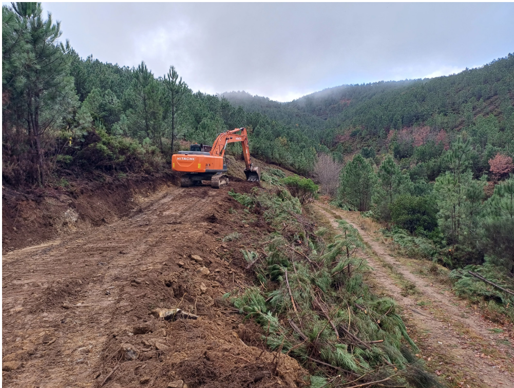
Figure 2. The plot of land carved with the company's excavator, November 16, 2023. Source: Mariana Riquito
